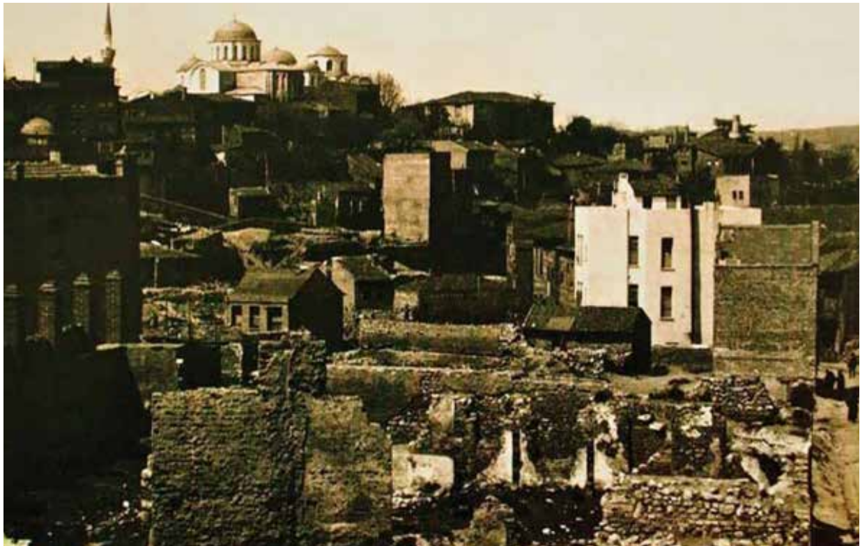
Figure 9. Zeyrek after fire
